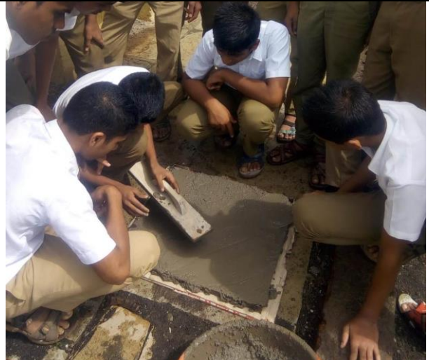
Chas IBT : Making ferrocement sheet
