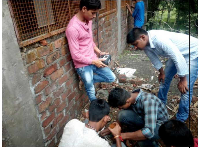
Making and testing earthing for new hostel
