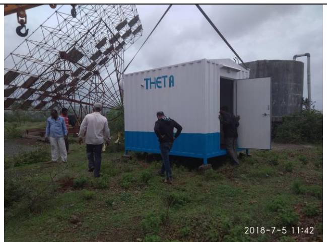
Heliostat getting installed at Pabal
