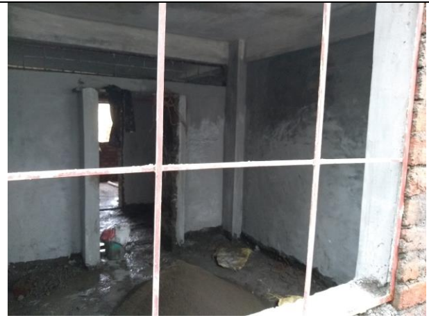
Status of new hostel room
