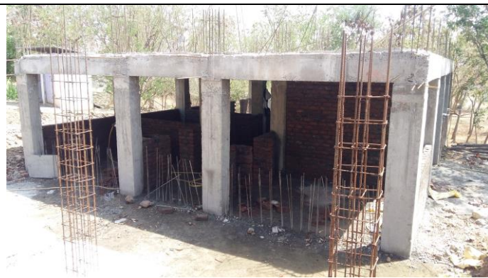
Status of hostel construction
