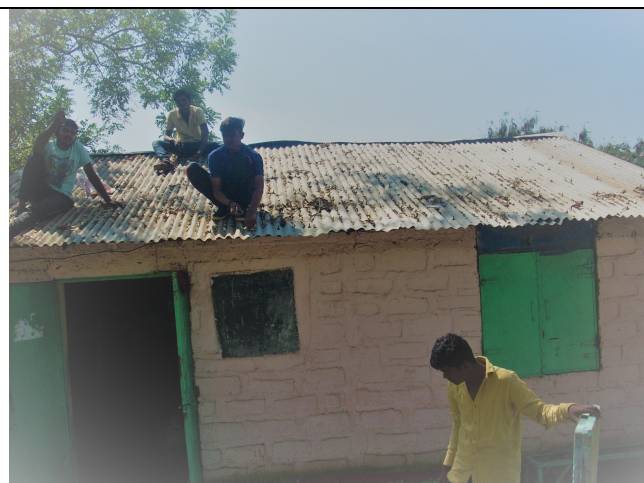
Hostel no.2 : Before getting demolished for new hostel
