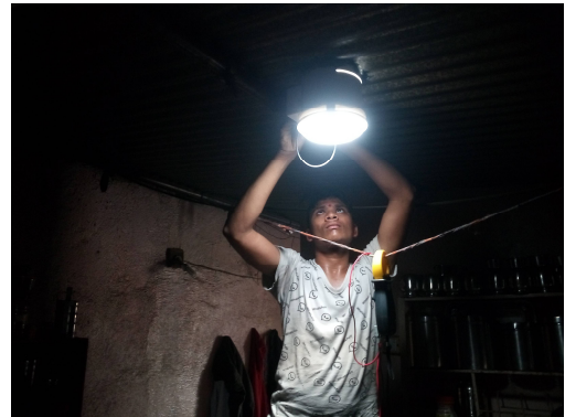
Installation of Micro Solar Dome
