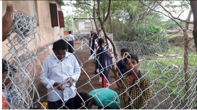
Students doing compound in Aichale IBT school
