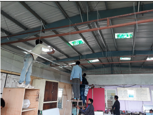
Students working on Falls ceiling of Electric Lab
