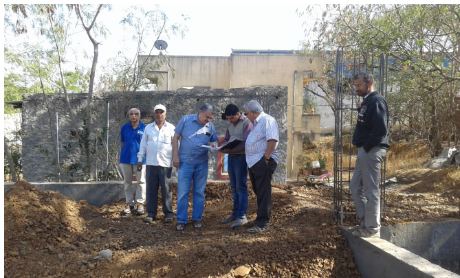
VA-MC members inspecting classroom construction
