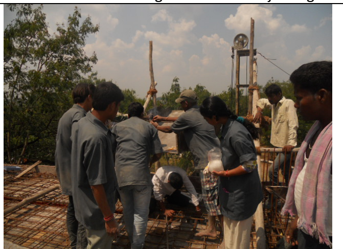
DBRT students working on kitchen slab work
