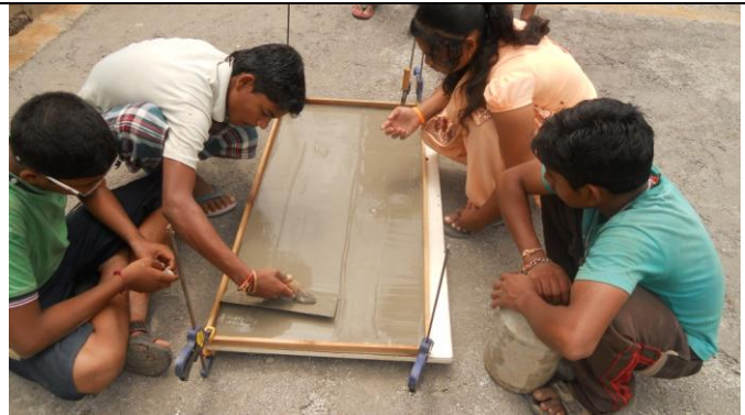
Making Ferro cement mould for kitchen wall
