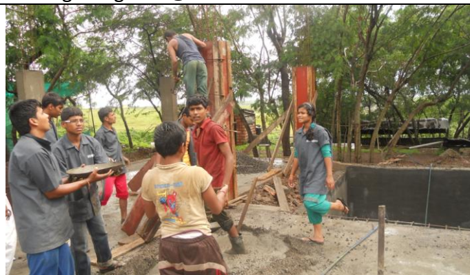
Kitchen construction in progress
