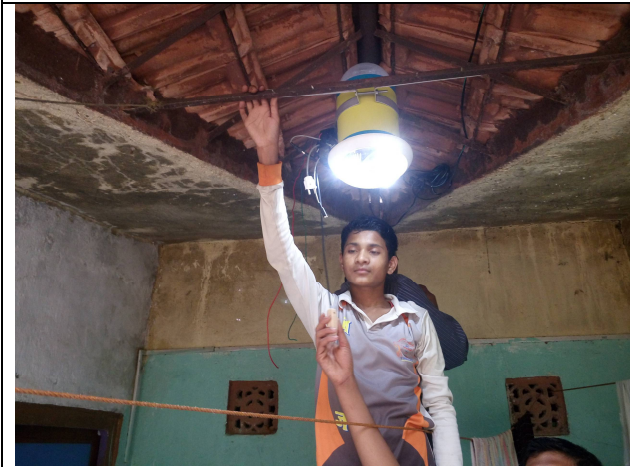
Installing micro Solar dome @ ashram
