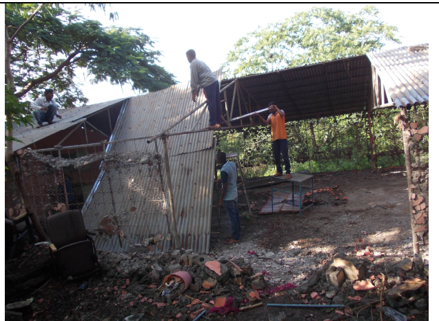
Demolition in progress
