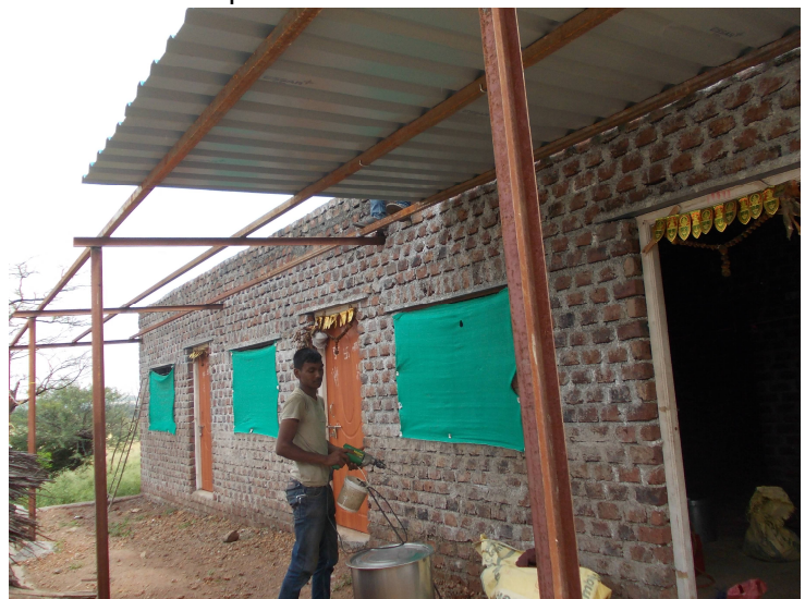
Shed in progress for school in Pabal
