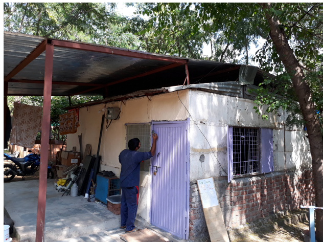
Renovation of staff quarter
