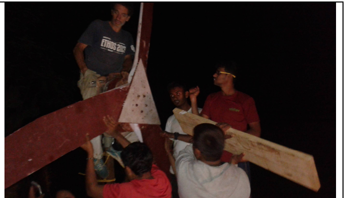
Installing wind mill at mid night on 29 th July
