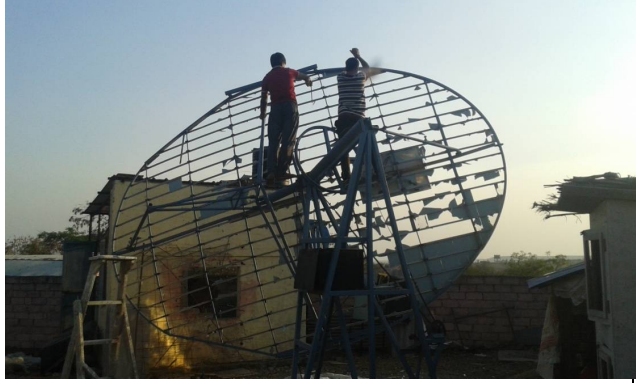
Retrofitting of glasses of Scheffler concentrator was done.
