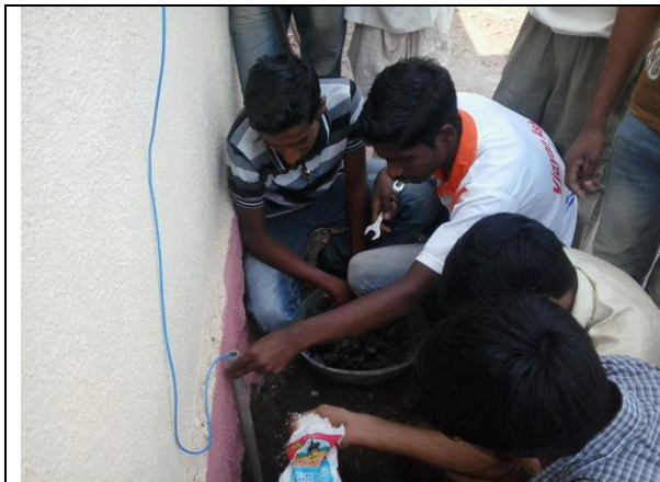
DBRT students carrying out earthing
