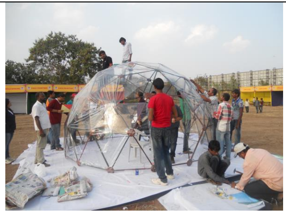
Erecting dome at Balewadi Sport complex
