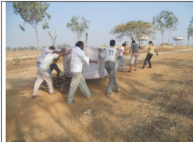
Shifting of water tank near plantation
