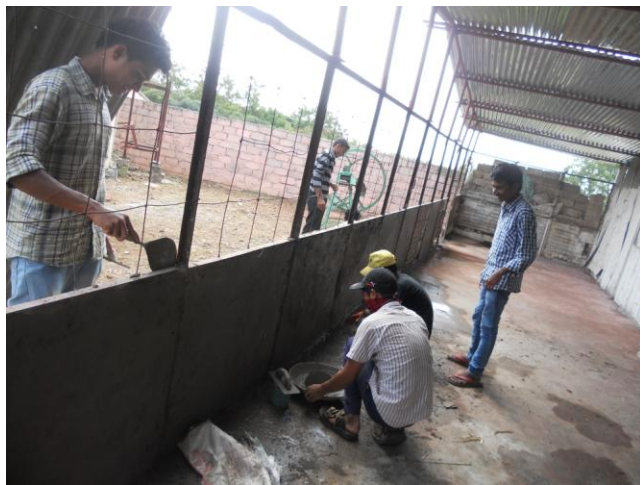
DBRT workshop students performing ferro-cement work
