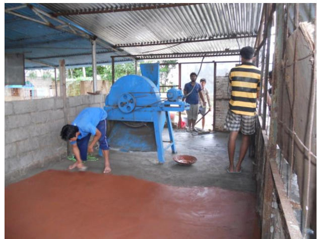
DBRT workshop students flooring work at cow shed
