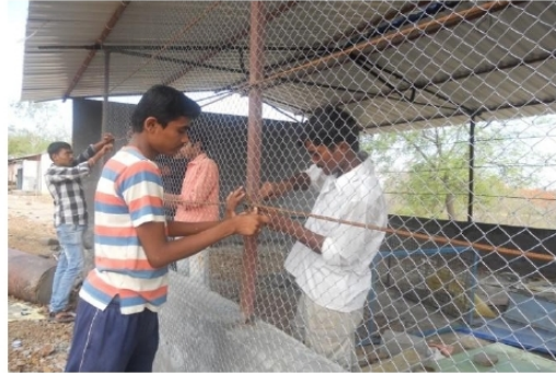
DBRT Students fixing chain link in newly constructed poultry shed.
