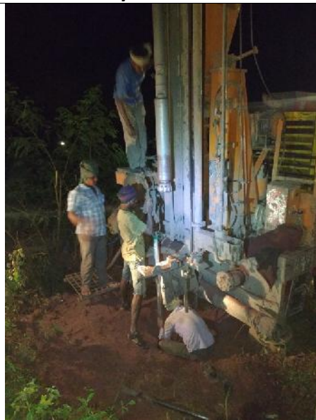
Boring machine made 10mtr drilling in the ground for earthing.
