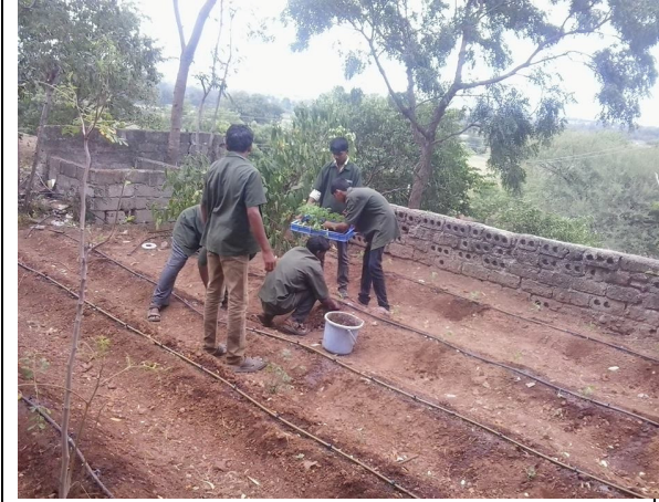
Installing drip and plantation @ ashram
