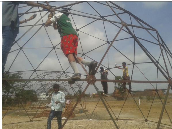
Dome construction @ Deepgruh
