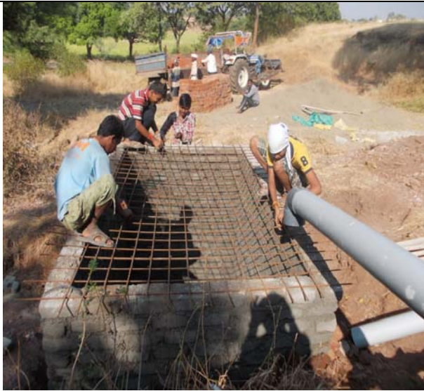
RCC practical on staff quarter's soakpit
