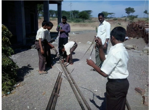
Walsang - IBT Doing welding work of Mr. Naik from village
