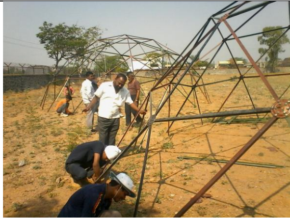
Dome construction at Deepgruh
