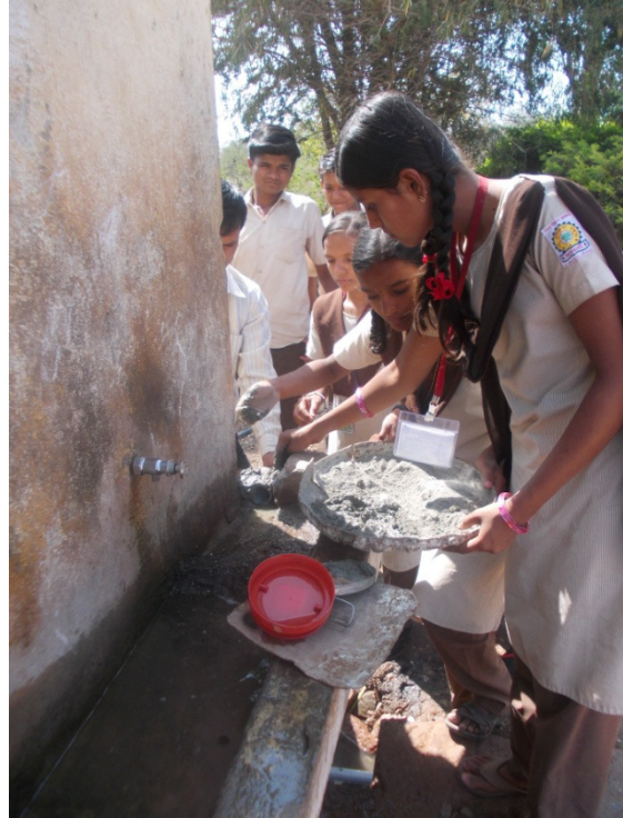
Construction practical :- Anavali school
