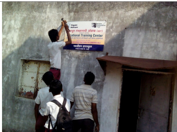
Installing IBT board in Patharai high school
