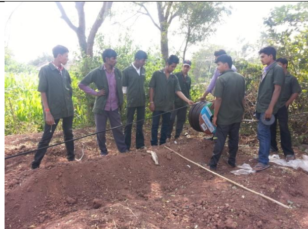
DBRT : Installing Drip at farmers field
