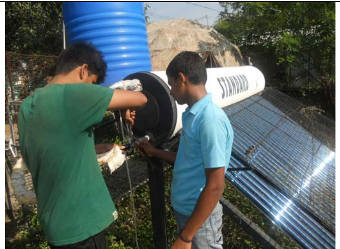
Fixing solar water heater
