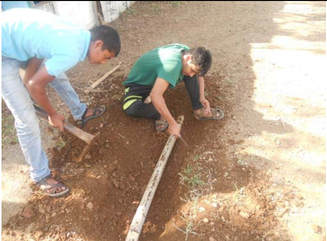
Carrying out piping job
