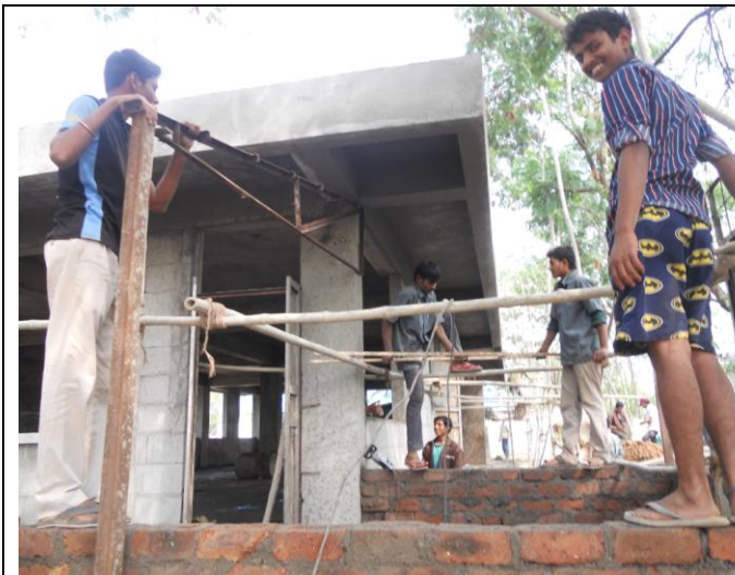
Construction of chulha shed
