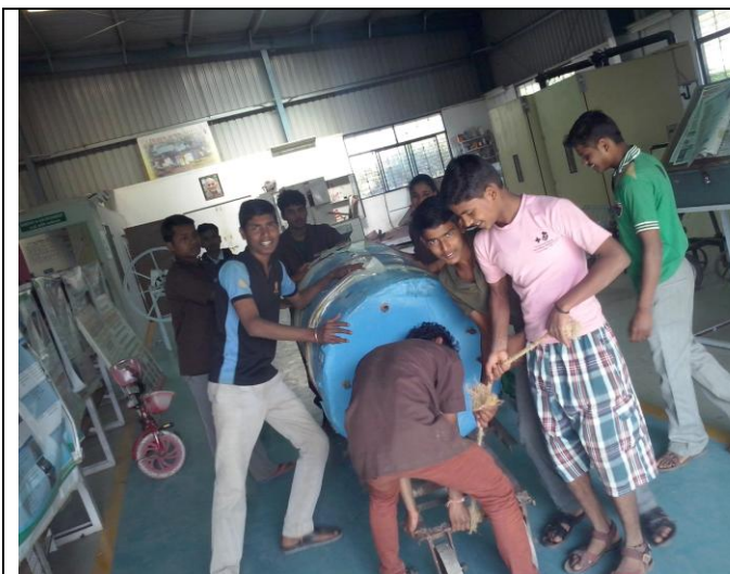
Repairing solar water heater @ workshop
